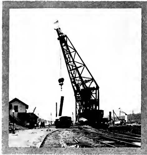
Fig. 6. The "Hercules" pulling up 6-foot caissons at the reloader wharf of one of the great coaling plants.
